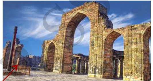
Made of Corbeled Arch Technique
